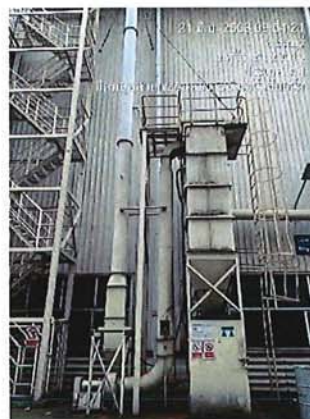
Dust Collector G.8 Forging 4
